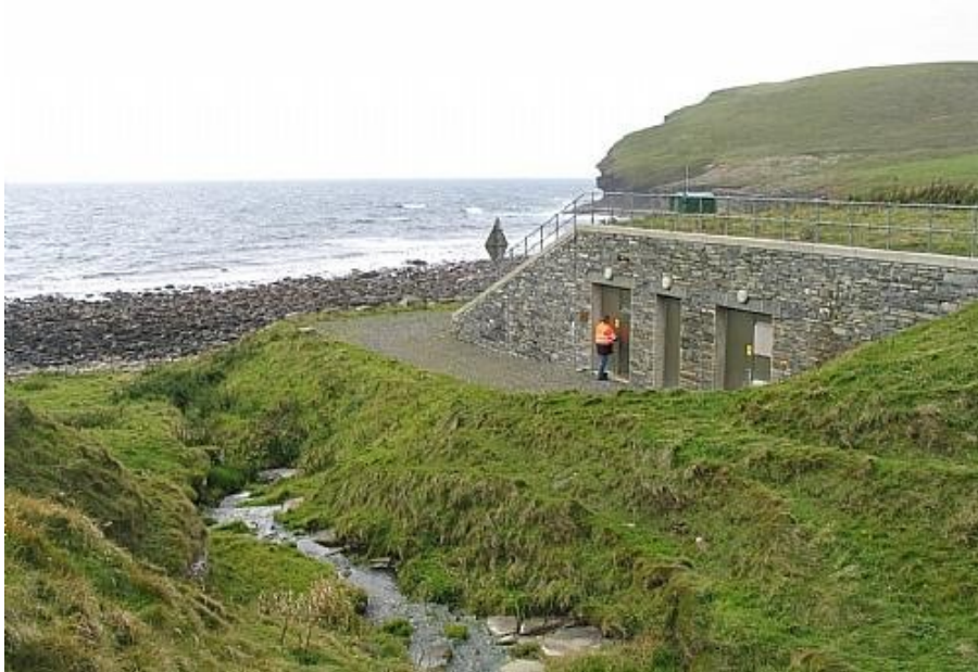
Figure 6: EMEC substation external view.
