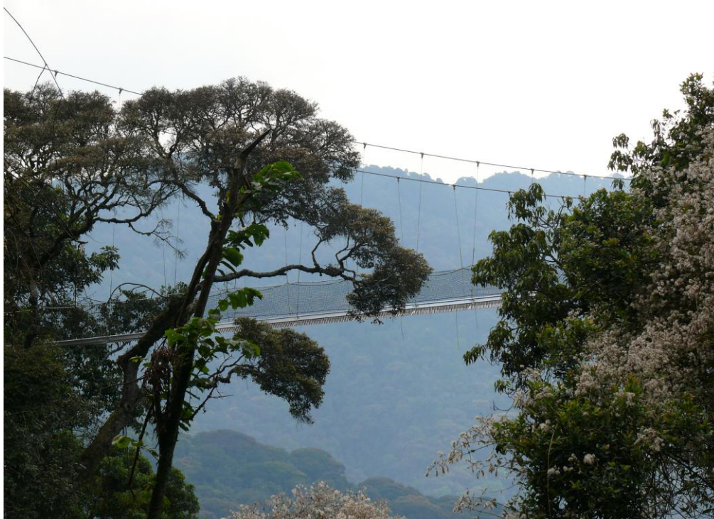
Picture 3: The Nyungwe canopy walkway in Rwanda was built by Greenheart Conservation Company Ltd. in 2010. The construction consists of three towers, three platforms and 165m of bridge connections.
