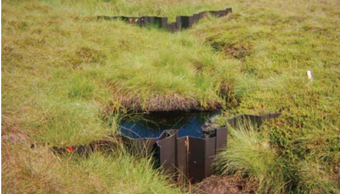
Figure 17: An example of drain blocking (Natural England, 2010).
