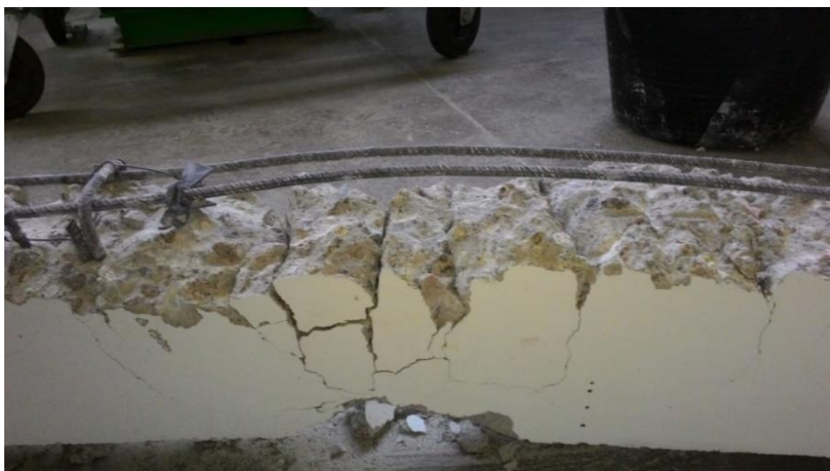
Photo 7: Beam B1 Yielded Tension Steel Bars.
