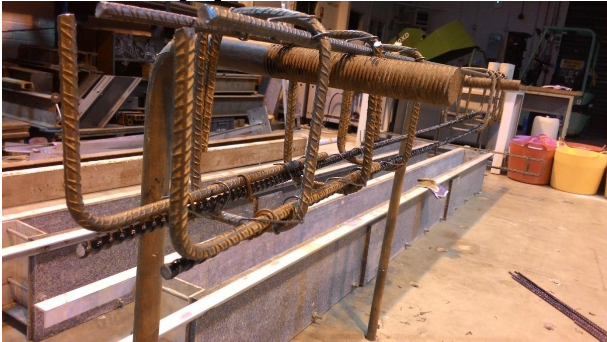
Photo 8 – BFRP and Steel Reinforcement Setup in Beams B2 and B4.
