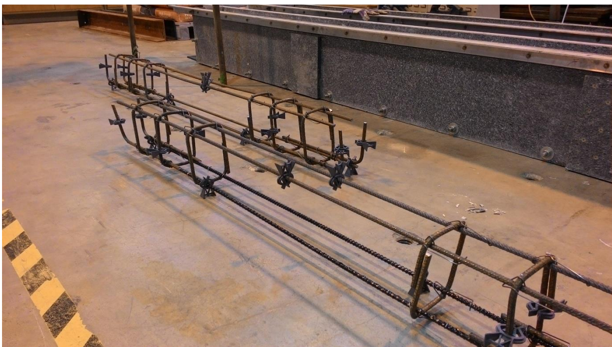
Photo 9 - BFRP and Steel Reinforcement Setup in Beams B1, B2 and B4
