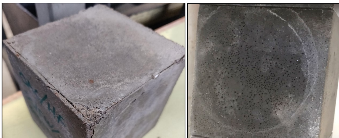
Figure 30: (left) - Without use of admixture Figure 31: (right) - Addition of admixture
