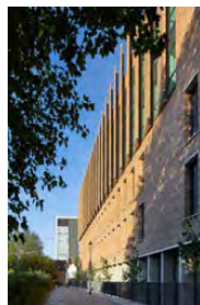
Figure 7: Exterior of AGB showing courtyard.
