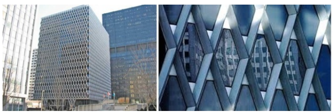
Figure 2: Integration of diagrid with the glazing system.
