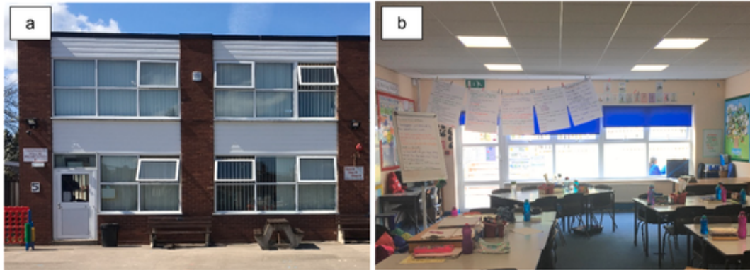
Fig. 4. Windows and external door in school 7, classroom 7.26 (a) and school 8, classroom 8.28 (b).
