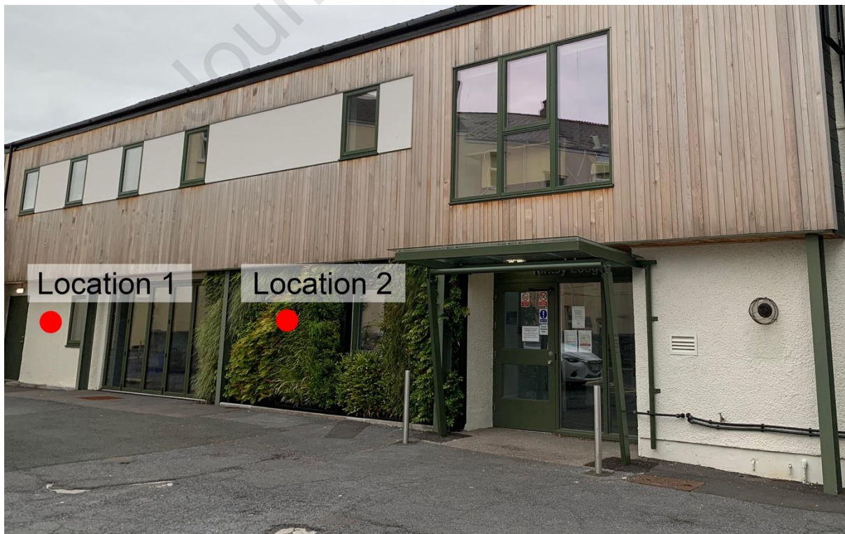
283 284 Figure 3. Photo of case study building, showing locations of monitoring setup.
