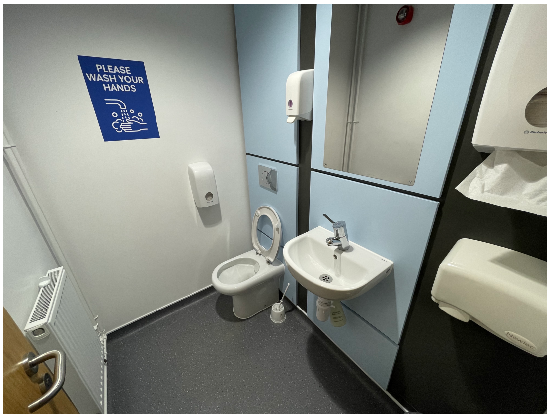
Figure 5.5: Representative toilet layout of site where sink traps 3 and 4 were located.
