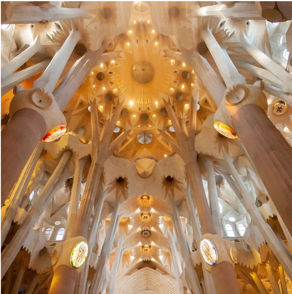
Figure 1: Sagrada Familia, biomimetic column (Kidd, 2019).
