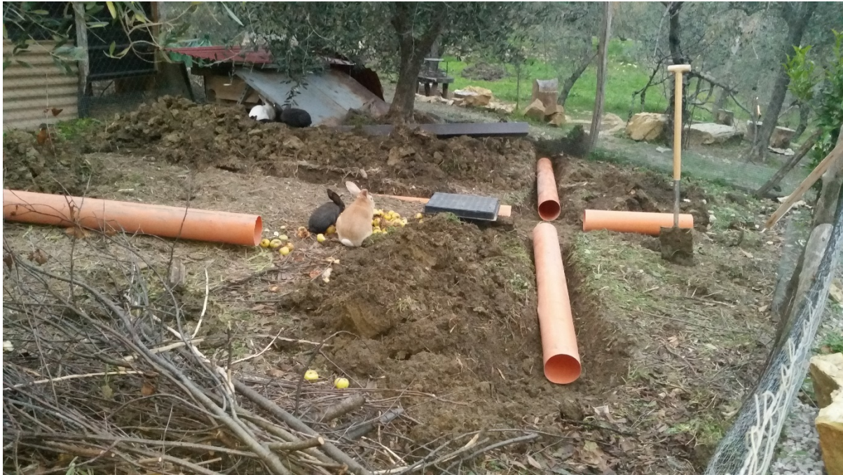
Figure 7.17 Building an underground tunnel system in the rabbit pen.
