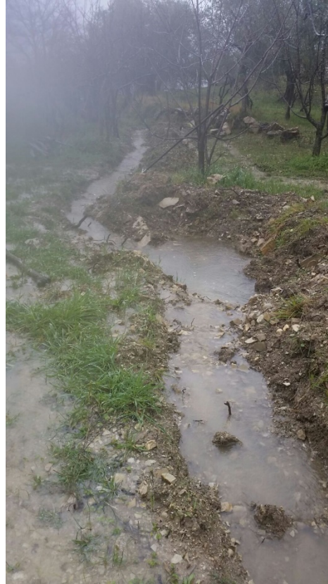
Figure 5.14: On the left: the land showing deep cracks and signs of salinization in the summer; and on the right: the land flooded in winter.
