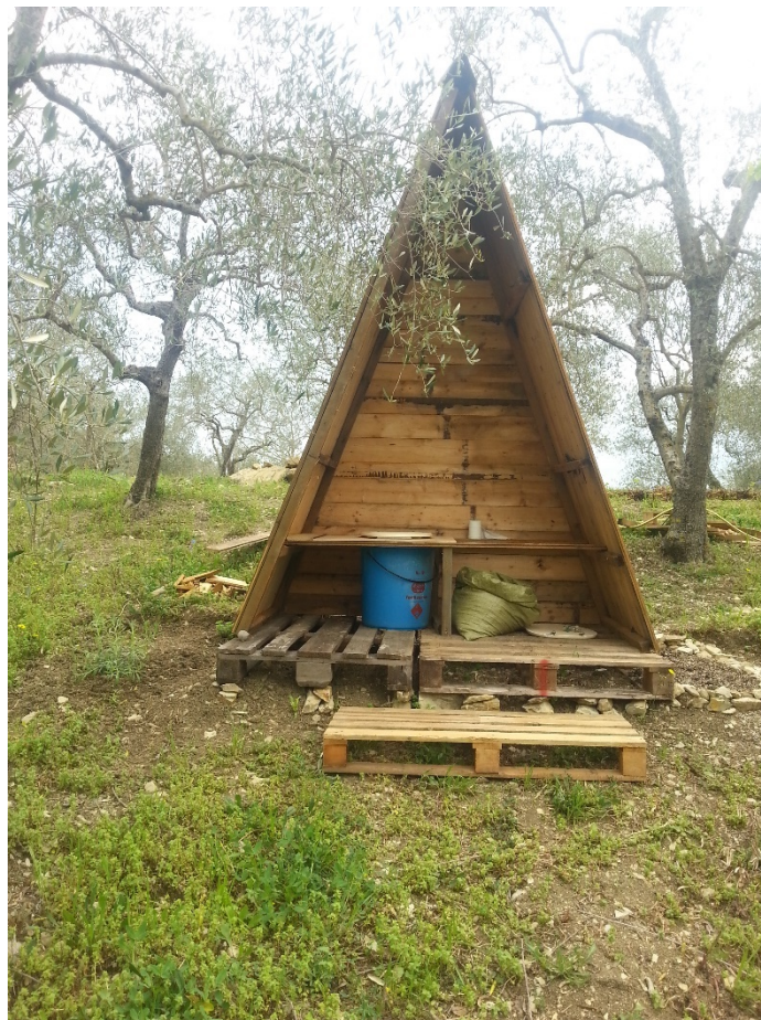
Figure 6.2 Our humble compost toilet.
