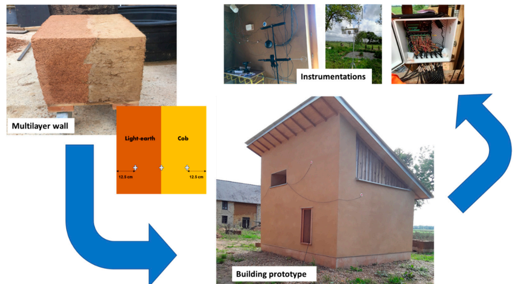
Figure 4. Description of the prototype building.
